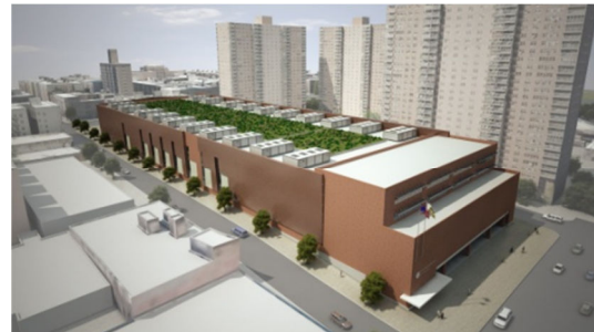
Figure 2: Rendering of the New York City Bus Depot showing its south face and both the corrugated metal and brick veneer facades. (Image courtesy of STV Inc.)
